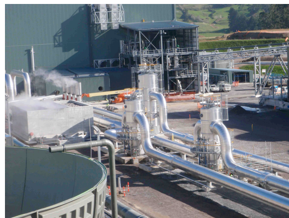
Figure 2.3.2: View of IP and LP Steam Scrubbers.
